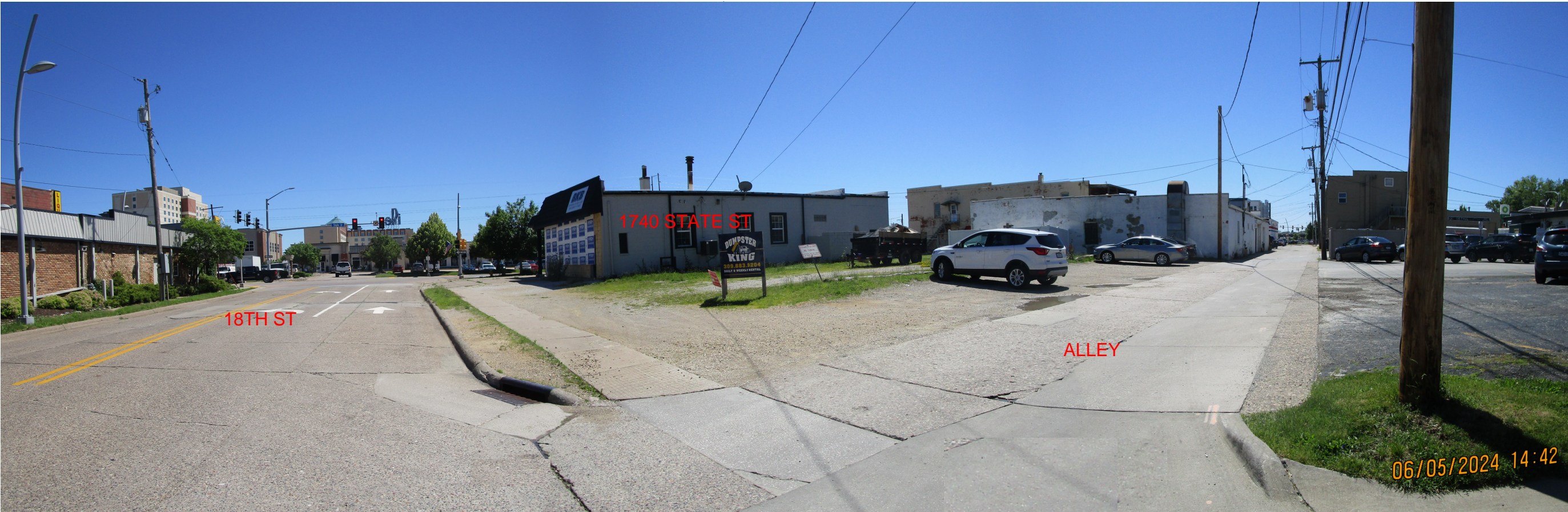
18TH STREET AND ALLEY LOOKING SOUTHWEST
